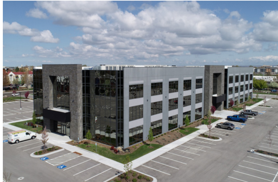
..... Above: Office Building in Silverstone business park, looking north-west.
