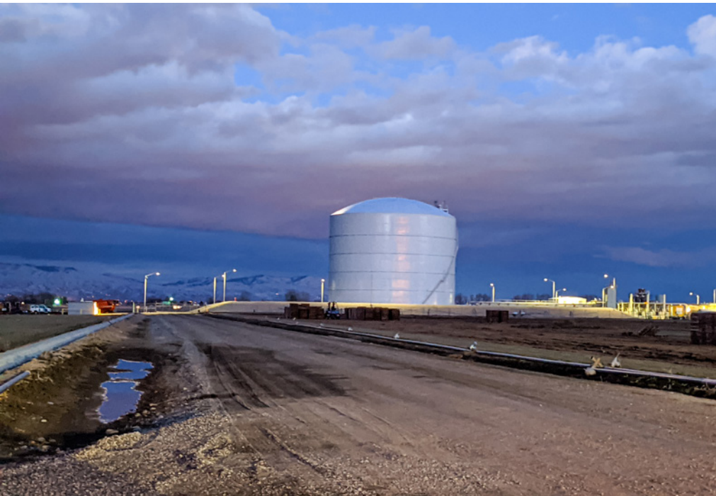
..... Above: Intermountain Liquefied Natural Gas Tank on Star Road, north of Ustick.
